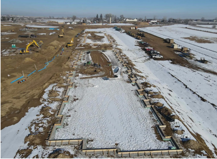
Apartments Phase 1 Construction
